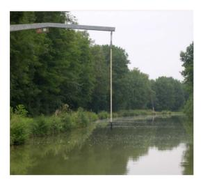
This pipe, requires a 'twist' of a quarter turn – you can hear it click as the circuit is 'made' -sending a signal to the lock, that the boat is there and ready to enter. The plastic pipe is soft, so you can run the boat under it and it won't damage your superstructure if it touches.
