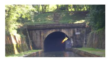
The long tunnel at *Pouilly* has an air height of 2.70 metres at its highest part, but be careful the tunnel roof is sharply curved. If your boat is a bit square, near the maximum height, I wouldn't risk it!
